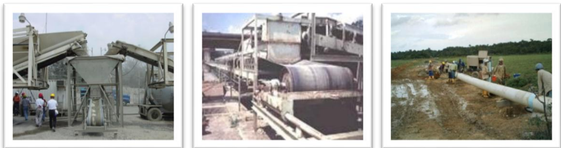
Figura tomada de: www.macoingenieria.com/images/montaje012.jpg
